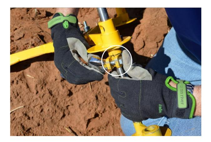
Re-tighten the nut and bolt (circled).
