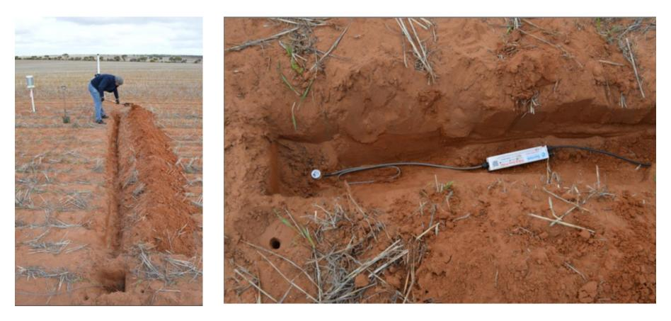
The entire cable is placed in a 20cm deep trench to protect it from cultivation tynes.
